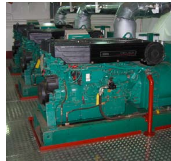
A multi-set installation with Volvo Penta D12 units providing electrical power on board a seagoing tanker.
